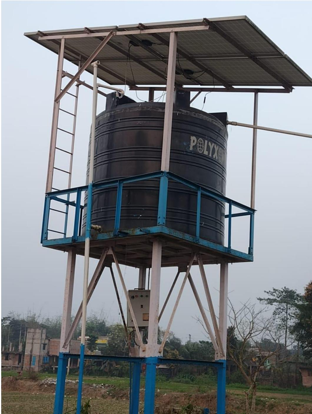
**Figure 3: Solar power based backup water pump, Siddhinath Mahavidyalaya**
